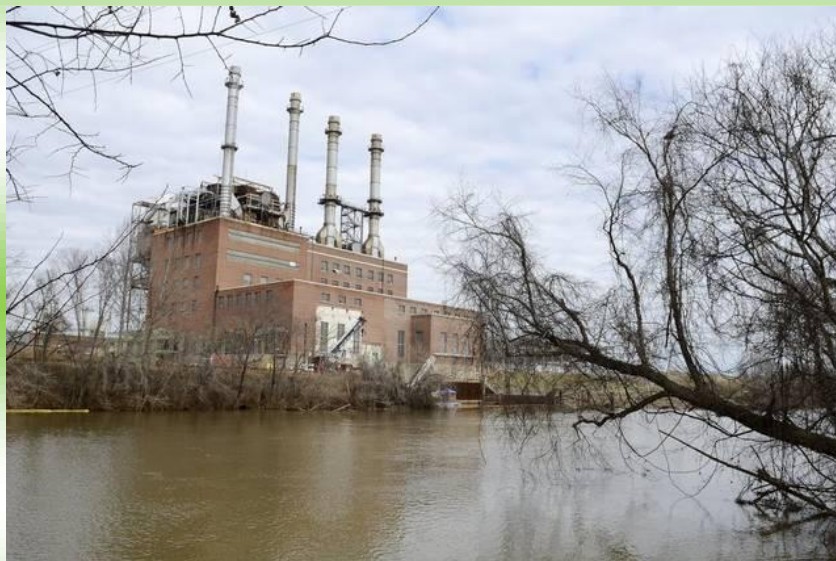
Duke Energy's Dan River Steam Station. (by: John D. Simmons jsimmons@charlotteobserver.com )
