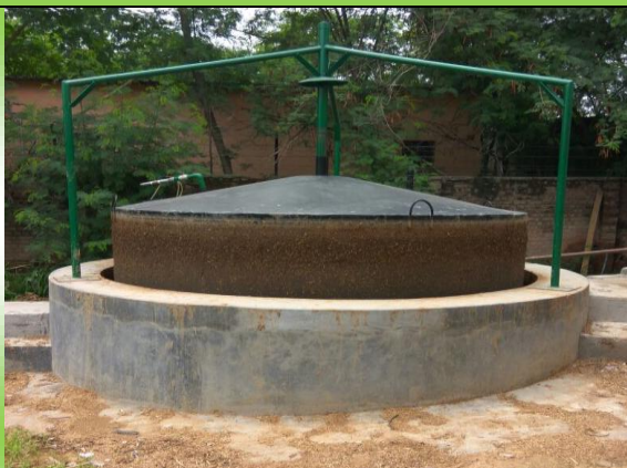
A 25 m3 biogas plant running from food/kitchen waste at IIT Delhi campus. Free dustbins distributed to residents of faculty apartment for in-house segregation of biodegradable and recyclable wastes- separately for making IIT Delhi campus clean and green, initiative taken in June 2016 by Prof. V.K. Vijay, Coordinator, Working Group on Waste Management, IIT Delhi.
